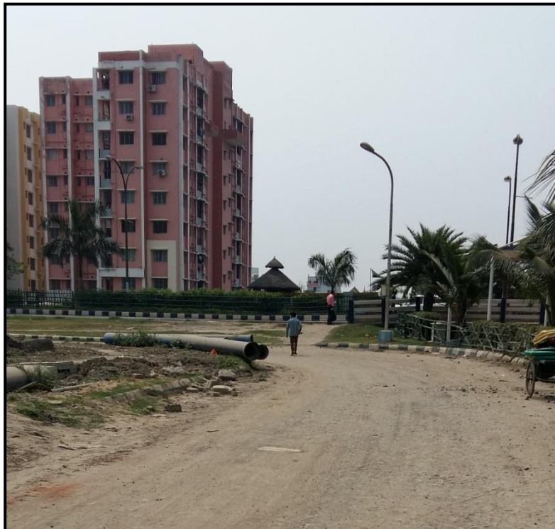
8. Location for Micro-tunneling Pit near bridge
