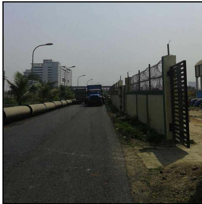
10. End of Transmission Line at BS-1
